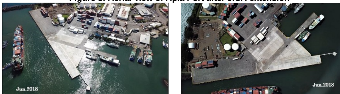
Figure 3: Aerial view of Apia Port after JICA extension
